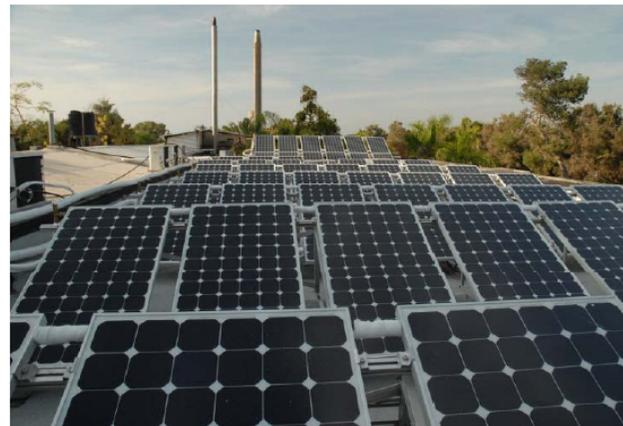
**\* Photovoltaic/Thermal = Rainbow uses water pipes to both cool PV panels and produce hot water**
