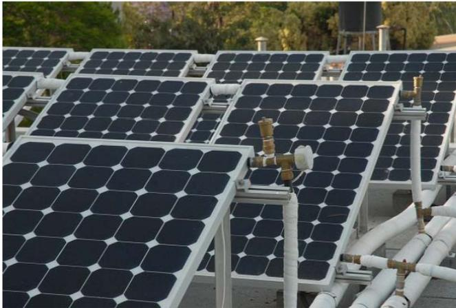
**PV/T panels with water temperature controller**
